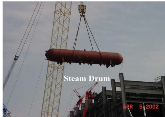
Fig 6. Erection of boiler drum
